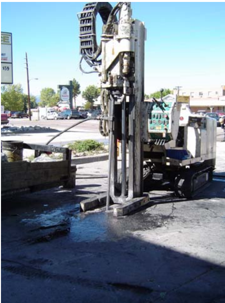
Site photo during injections
