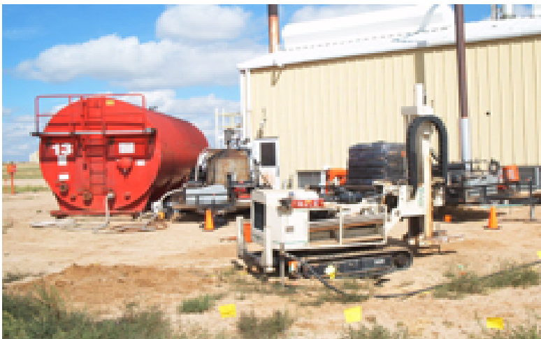
Site photo during injections
